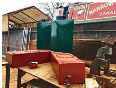
Rebottomed and painted diesel tanks
